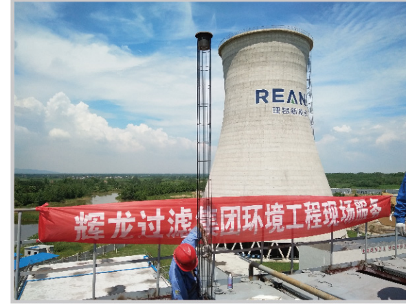
现场安装 Installation
